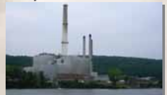
Nuclear Plant Protection
